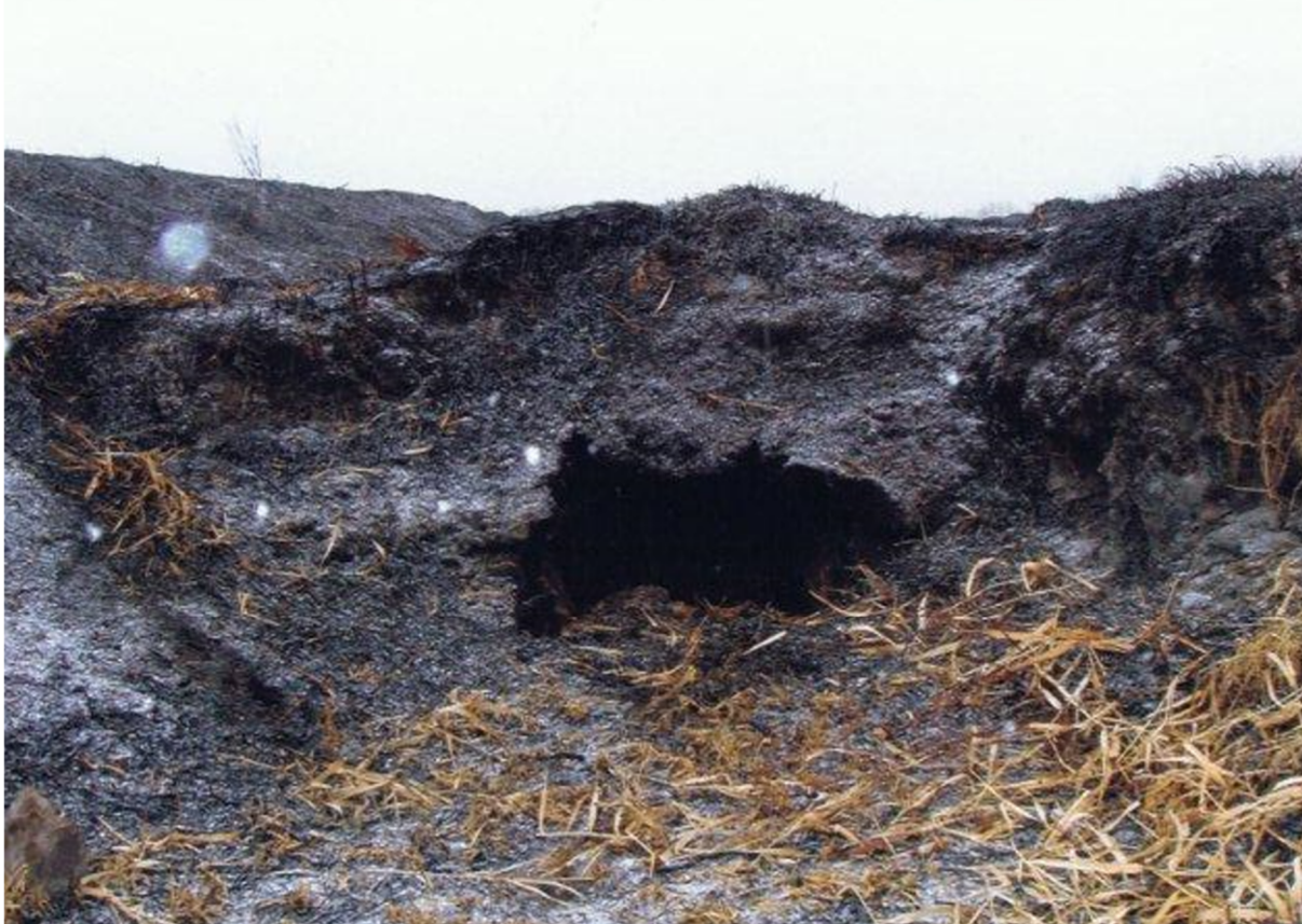
Figure 2. Sediment Covering the CD77 Mainline Tile Outlet
