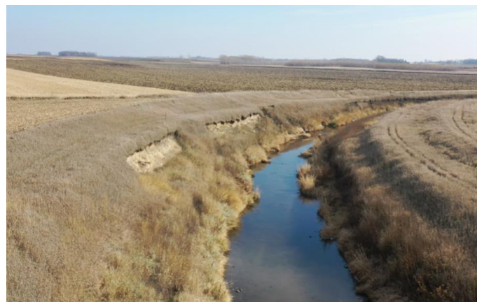
Picture #8: Sloughing along a bend in open ditch
