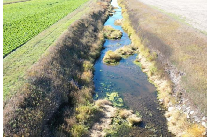
Picture #2: Vegetation growth in bottom of open ditch
