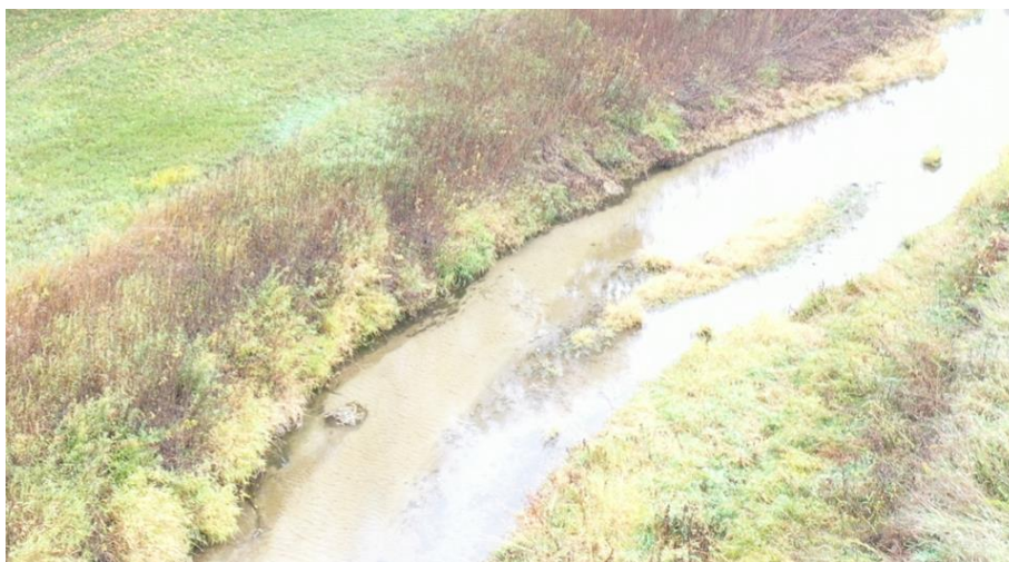
Figure 5: Sediment deposit in the bottom of the open ditch (NW ¼ of Section 12 of Wang Township))
