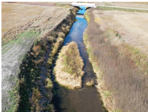
Picture #3: Slough around bend in open ditch with vegetation growth in bottom of ditch
