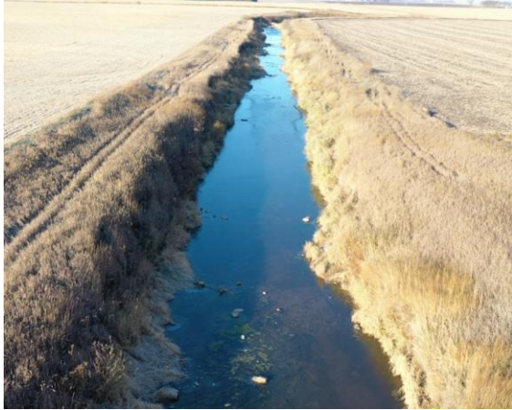
Picture #1: Major sloughing along left bank of open ditch
