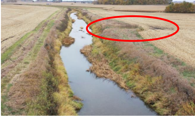
Picture #9: Visible erosion at potential ASI location (right)
