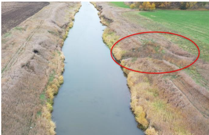
Picture #7: Gully erosion resulting in a washout on right side of open ditch
