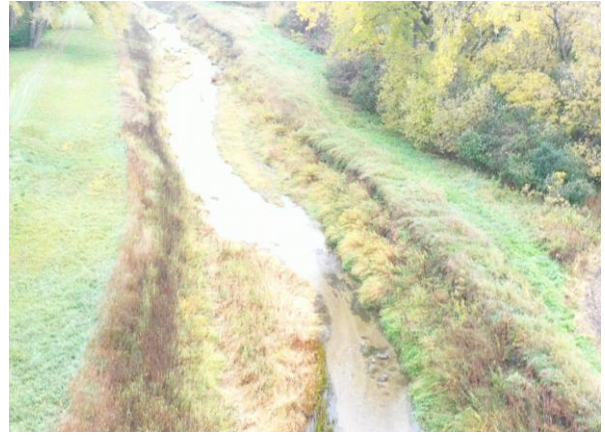
Picture #6: Sediment accumulation in bottom of open ditch
