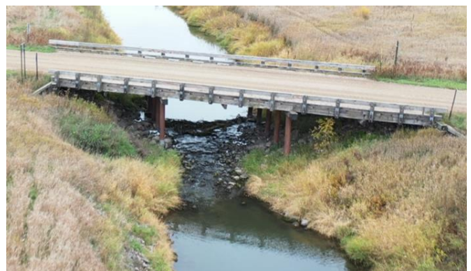
Picture #4: Sediment accumulation under bridge along 880 th Ave
