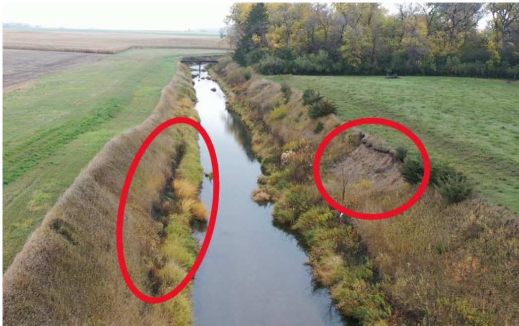
Figure 3: Isolated sloughing shown in the red circles (SW \frac{1}{4} of Section 14 of Ericson Township)
