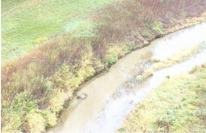
Picture #5: Sediment accumulation in bottom of open ditch
