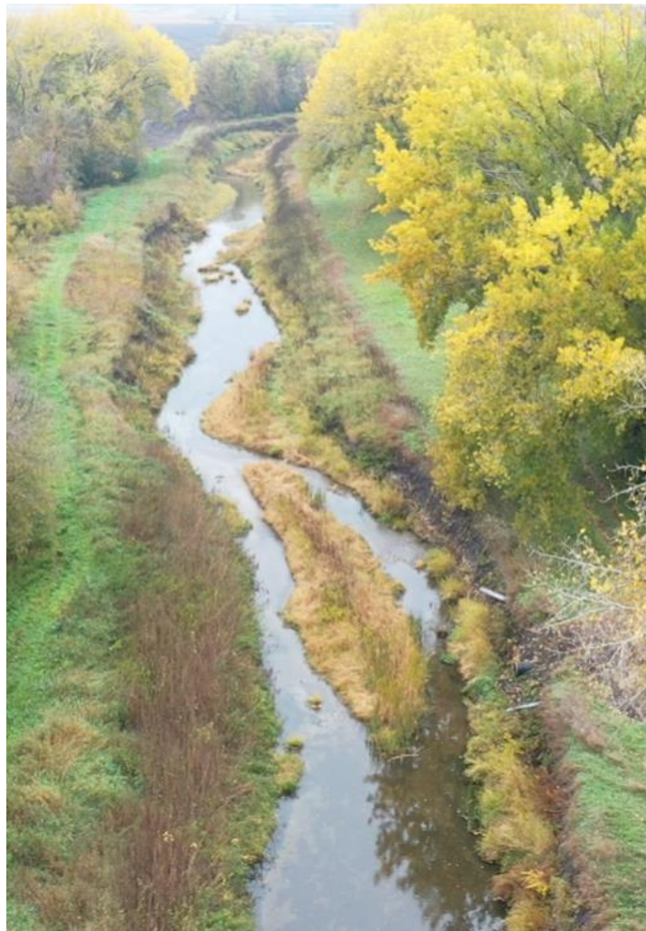
Figure 4: Vegetation growing within the bottom of the open ditch (NE ¼ of Section 12 of Wang Township))
