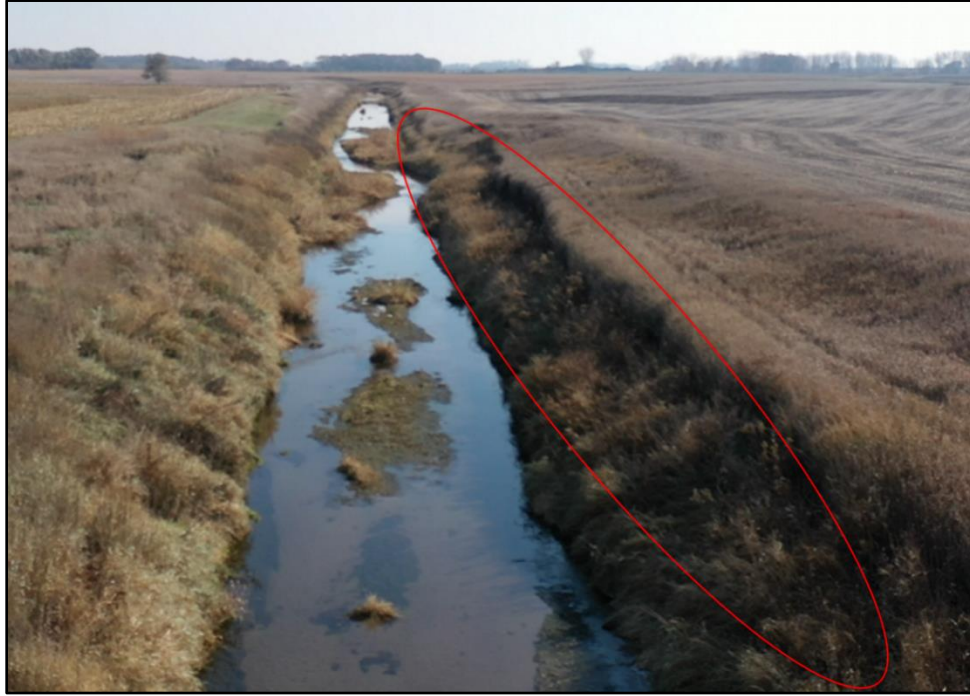
Figure 2: Bank sloughing along the right side of the open ditch (SW \frac{1}{4} of Section 15 of Ericson Township)
