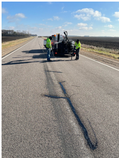
Photos Above: Crack Filling Co. Rd 11 West of Co. Rd 5
