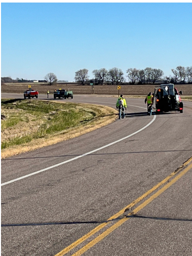
Photos Above: Crack Filling Co. Rd 11 West of Co. Rd 5
