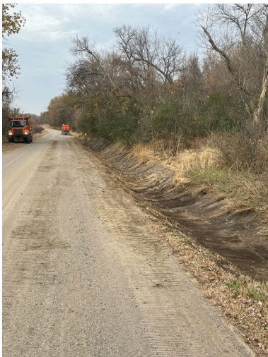
Photos Above: Co. Rd 51 Ditch Cleaning
