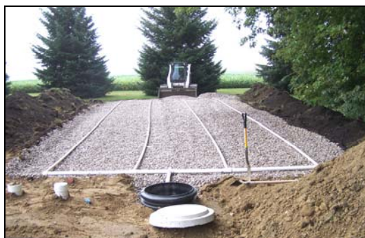
Photo: Installation of a septic drainfield.
