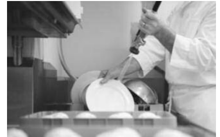
Upgrading to a more efficient pre-rinse spray valve can decrease the amount of water needed to rinse dishes.
