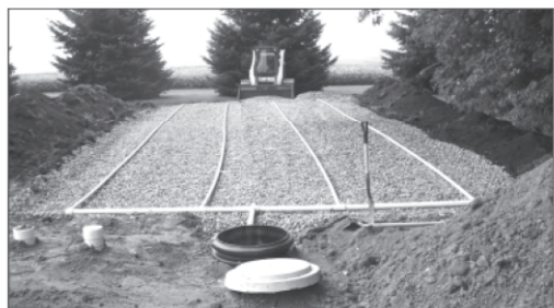
Installation of a septic system drainfield.
