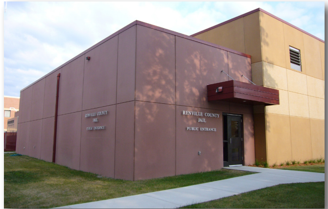
Renville County Jail Public Entrance
