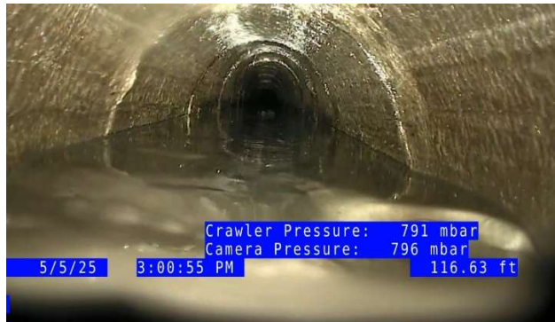
Image 2: Br Main B 14" filled with sand. Parcel Number 11-00390-00
